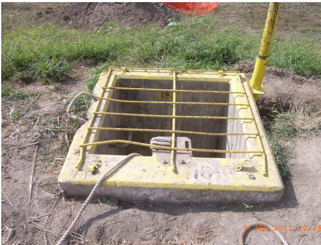
Photo 2- Gatewell Structure, at the time O&M staff cleaning structure and install new sluice gate
