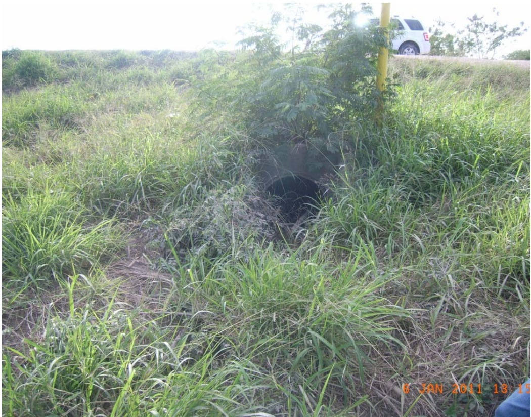
Photo 2- Landside inlet, to be cleaned and vegetation to be removed.
