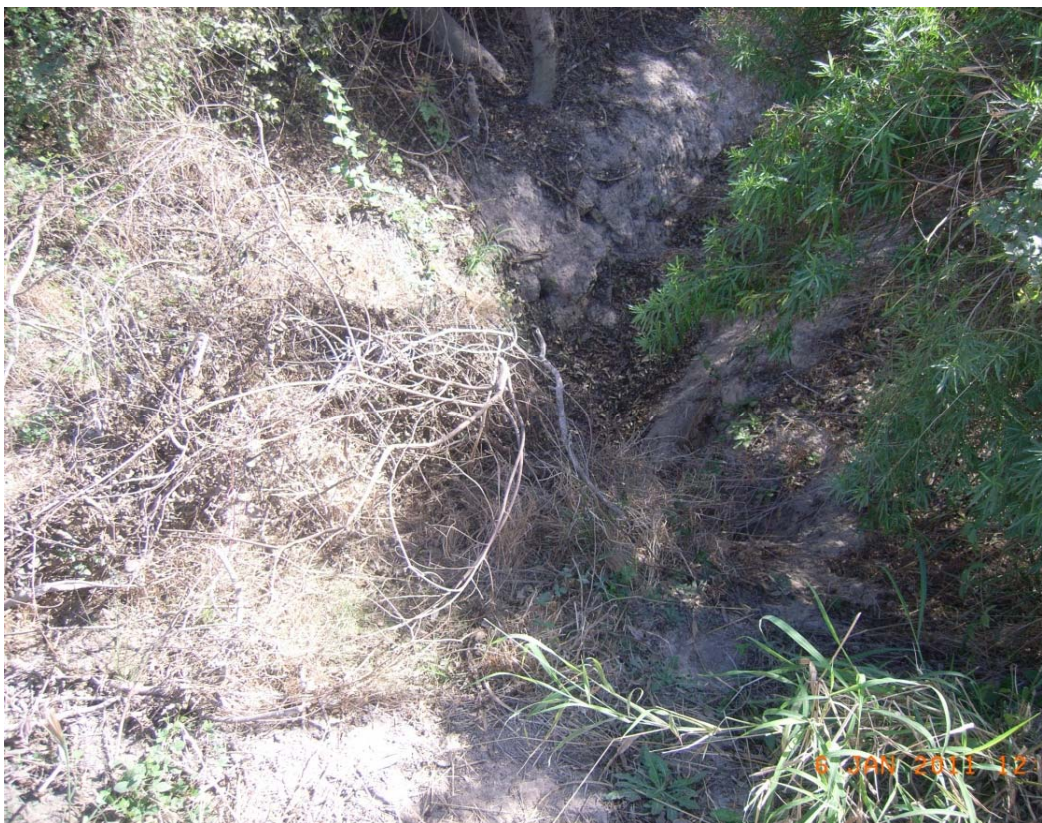
Photo 2- Riverside Inlet Ditch with debris and vegetation.
