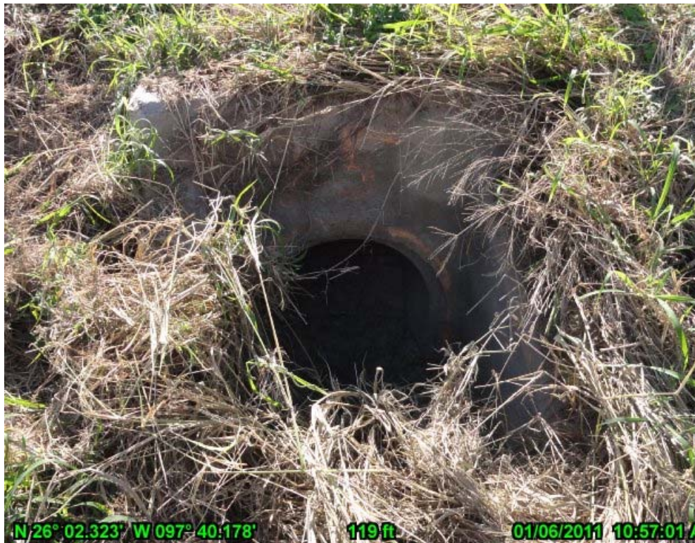
Photo 2- Riverside Inlet, to be cleaned and remove vegetation
