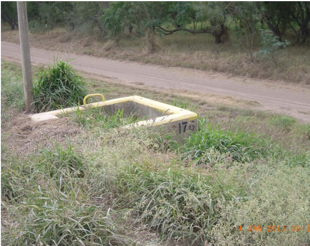
Photo 1- Gatewell Structure 176, abandoned
