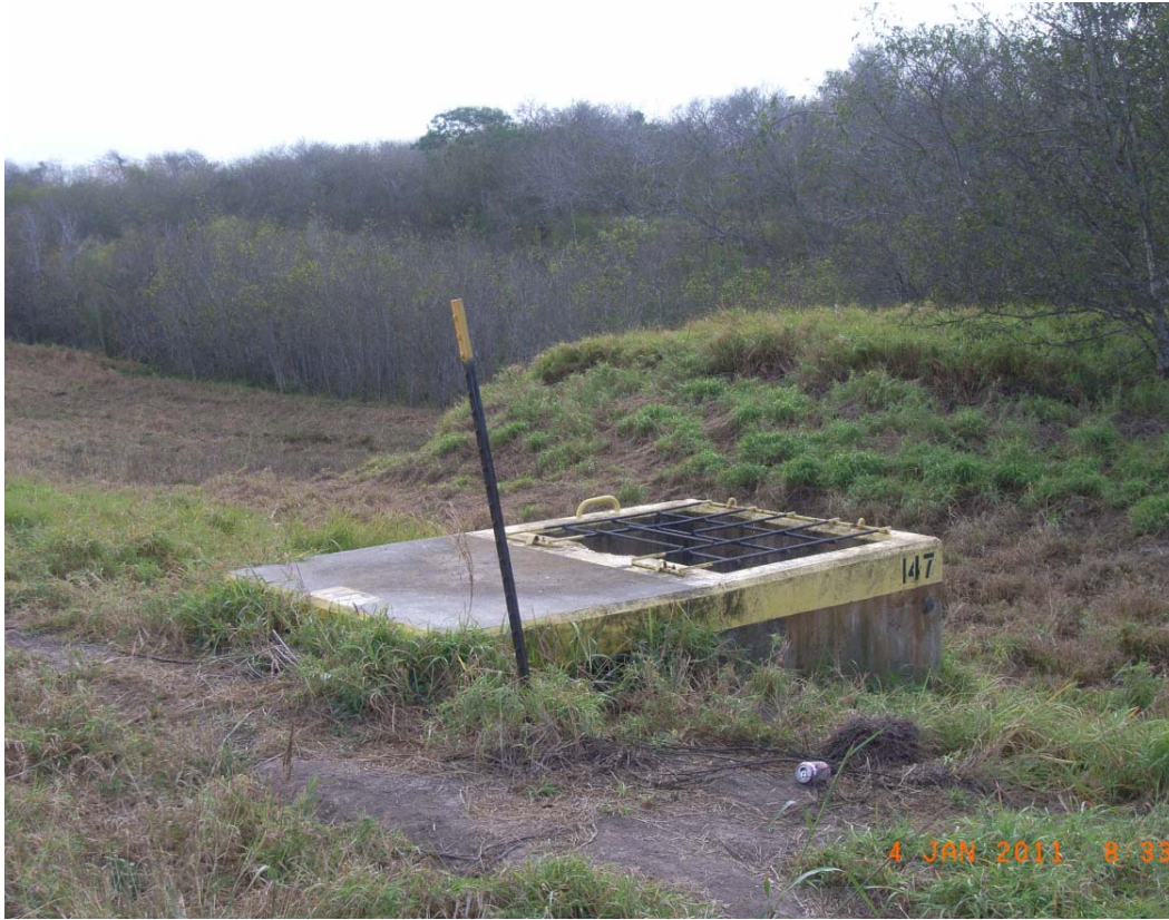
Photo 1- Gatewell Structure 147, missing top of sluice gate
