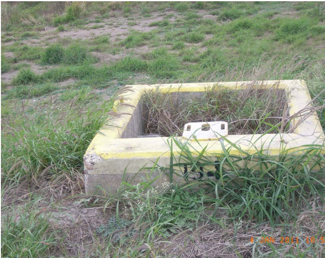
Photo 1- Gatewell Structure 194, abandoned
