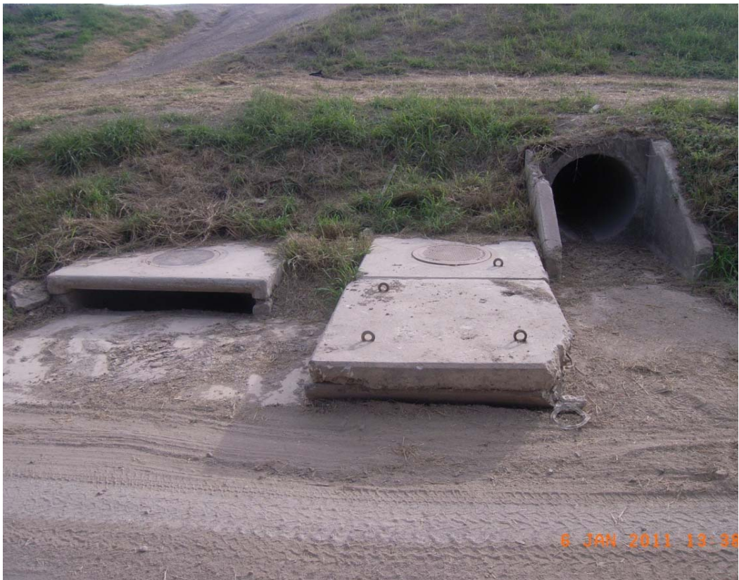
Photo 2- Landside inlet structure
