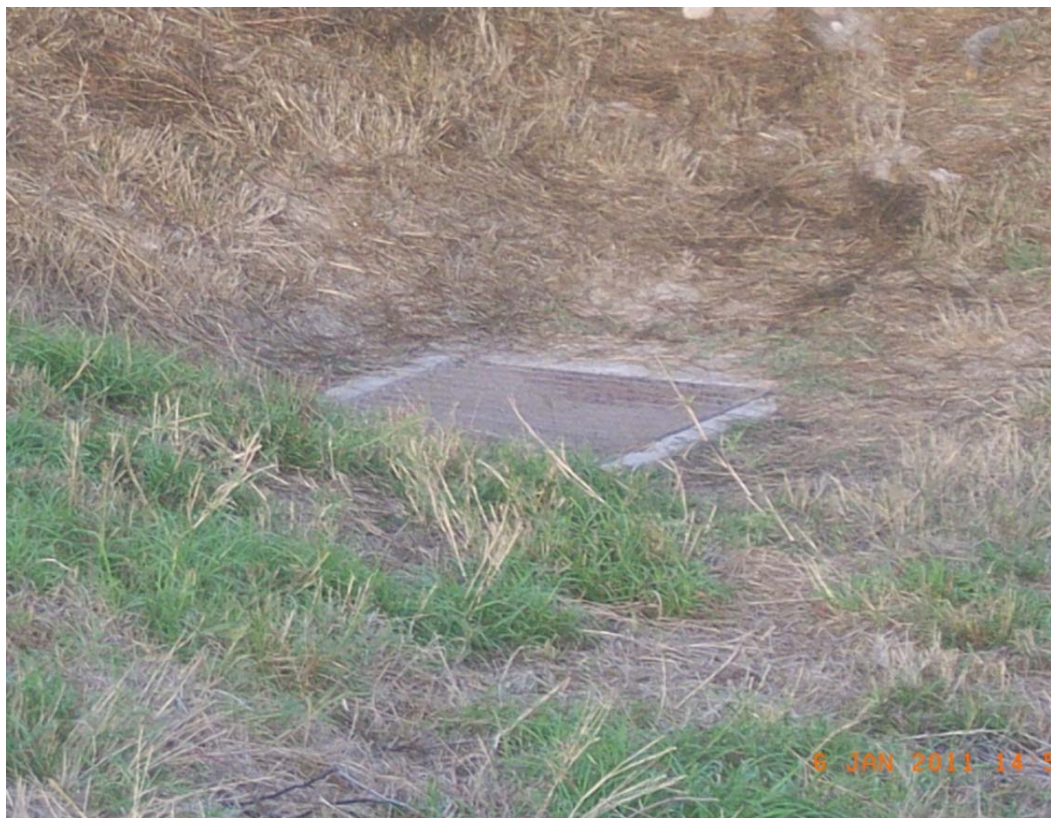
Photo 2- Landside inlet at bottom of slope.
