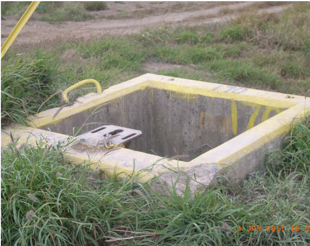
Photo 1- Gatewell Structure 170, abandoned
