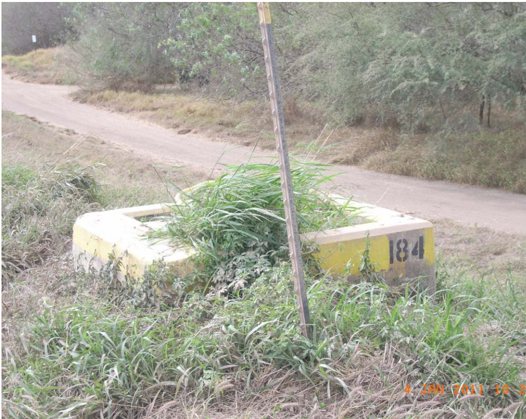
Photo 1- Gatewell Structure 184, abandoned
