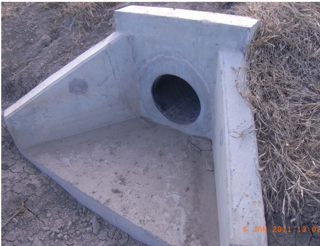
Photo 2- Landside outlet structure
