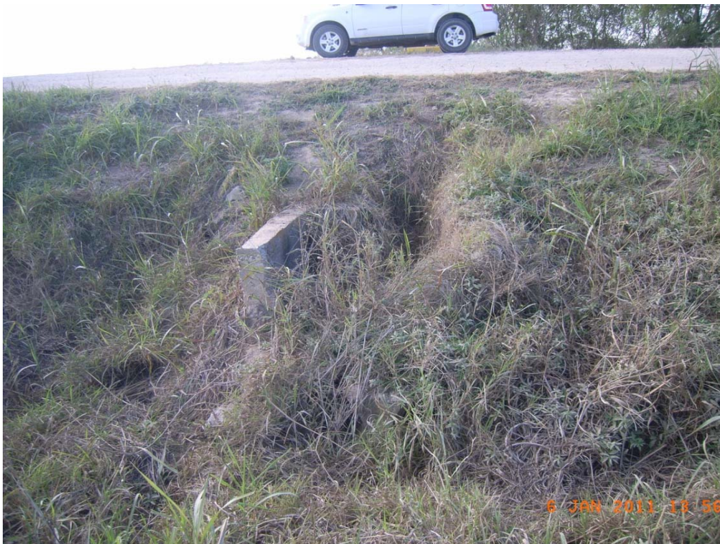
Photo 2- Landside inlet, to be cleaned and remove vegetation
